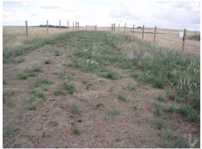
Fig. 3 Pipeline July 2006 following hay application
